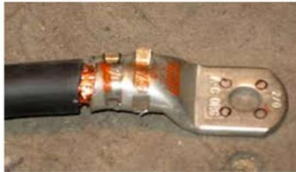
Prepare wire and terminate with crimped terminal lug as shown to fit M10 bolt screw. Use the included M10 hardware to fix to the busbar.
